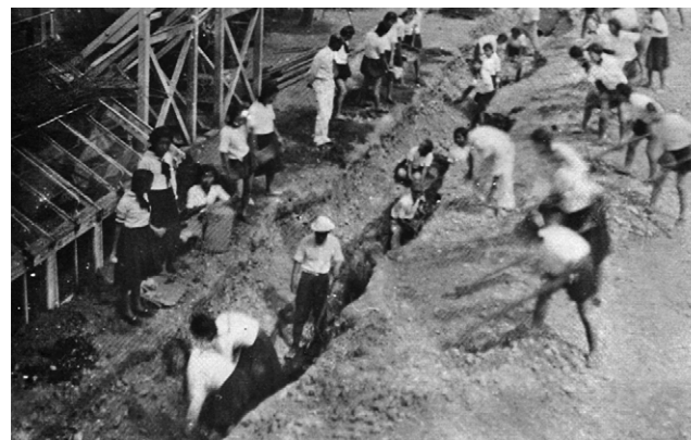
防空壕を掘る富田高女生
